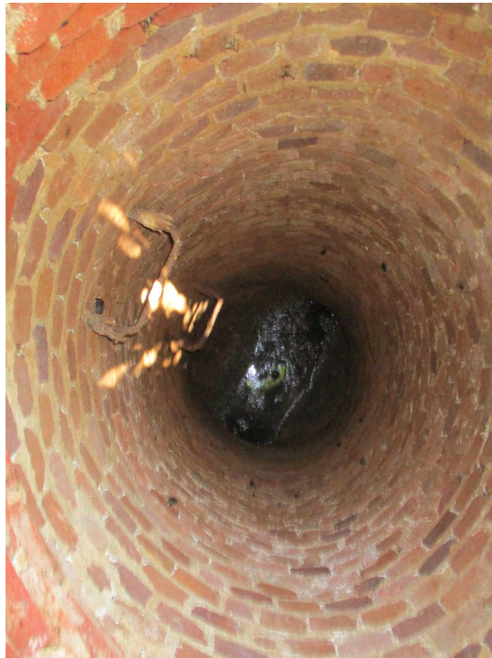
Brick manhole in front of Commonwealth Attorney's office.
