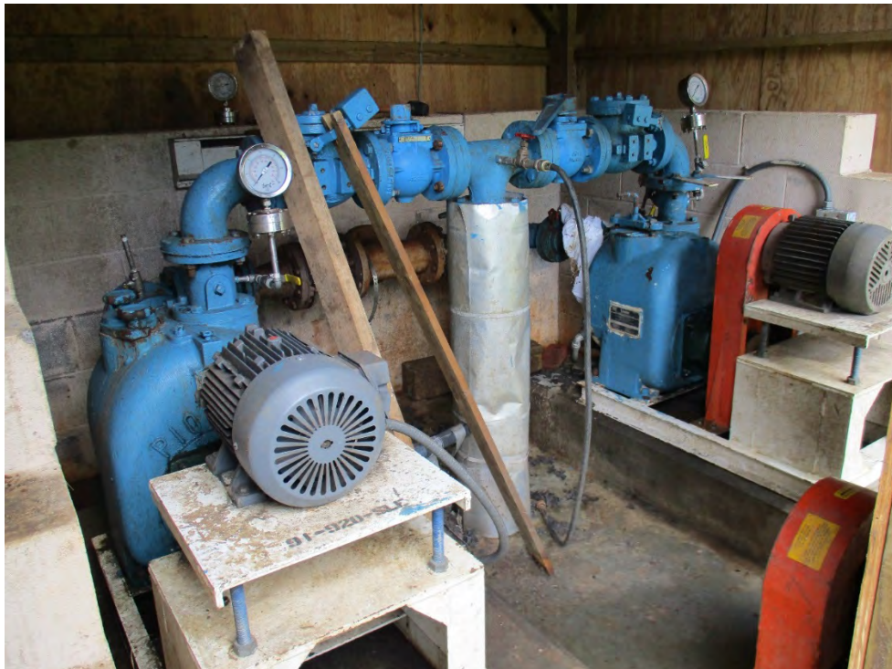
This is an image of the return sludge pumps. Both pumps have been recently refurbished and there is one on standby.
