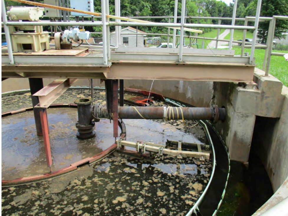
This image is of the clarifier at the Drakes Branch WWTP. The drive for the clarifier has been recently replaced.
