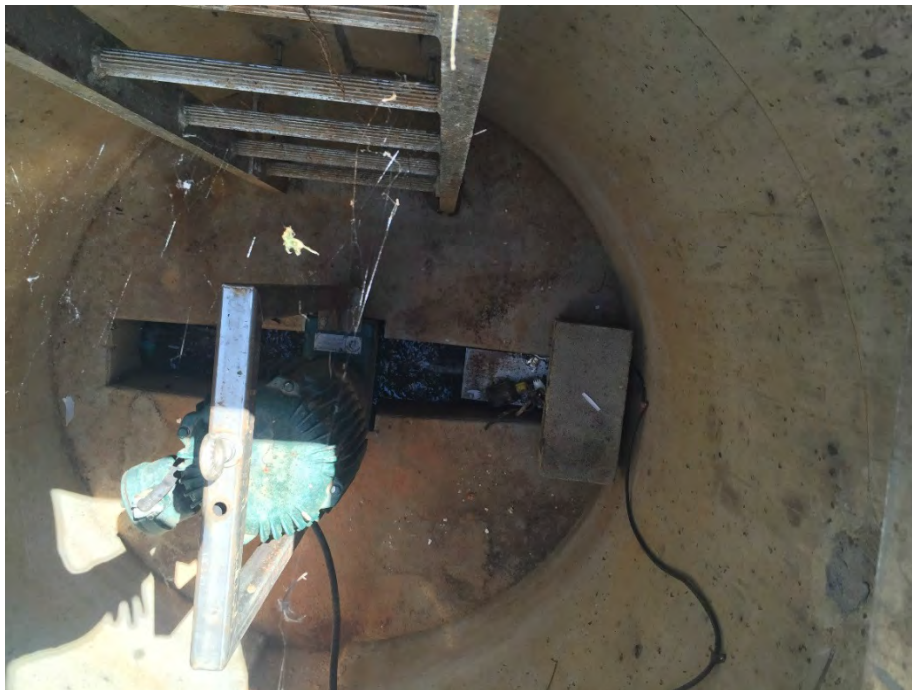
Comminutor Grinder at the Administration Building Pump Station.
