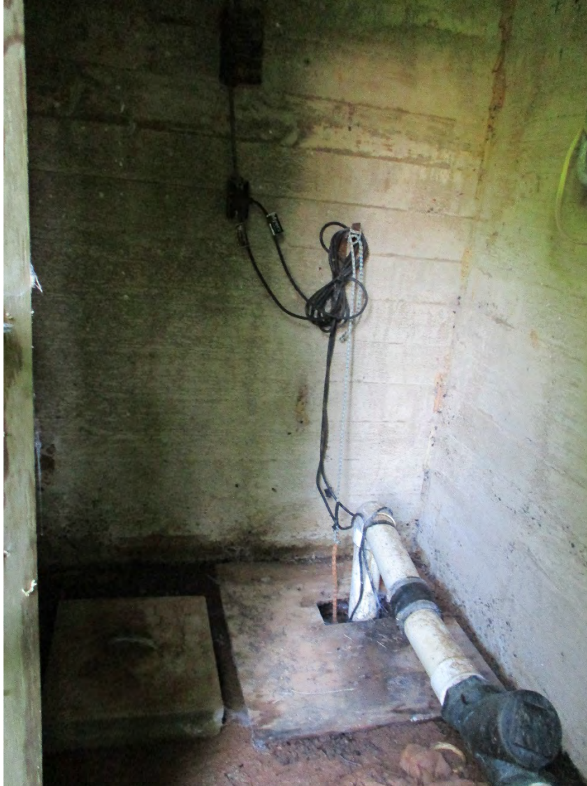
The forcemain leaving the wet well of the Health Department Pump Station inside the pump house.
